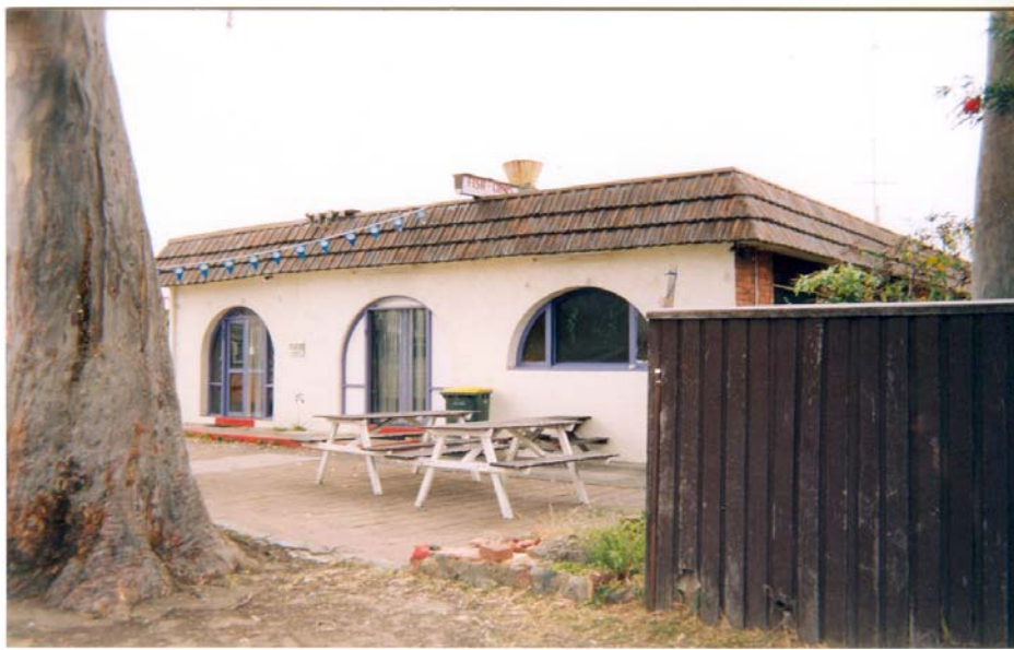
PHOTO 5.1: Closed takeaway food establishment, Tarean St.
