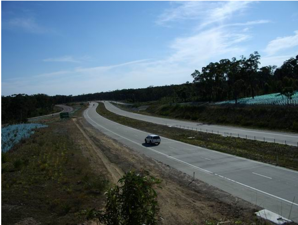
Photo 2.1: The bypass data collection point
