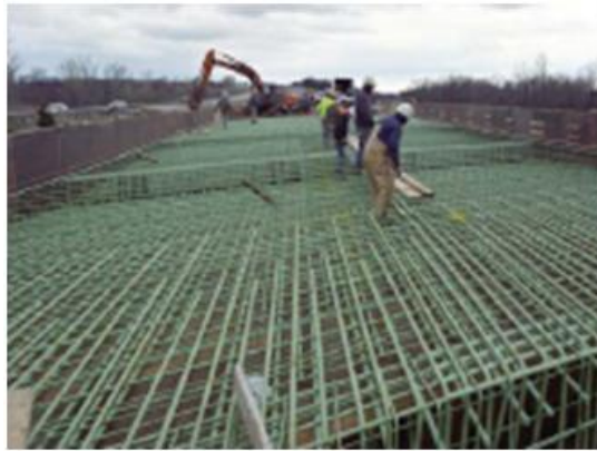
Bridge Deck Replacement
