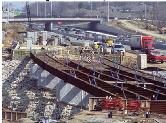
Bridge Structure Replacement
